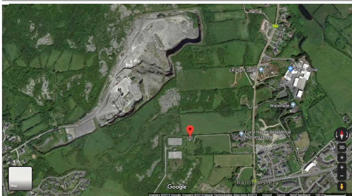
Figure 1: The location of the communications tower (ITM 530660 728015) which would be suitable for the placement of a nest box for Peregrine (shown by the red pin).
